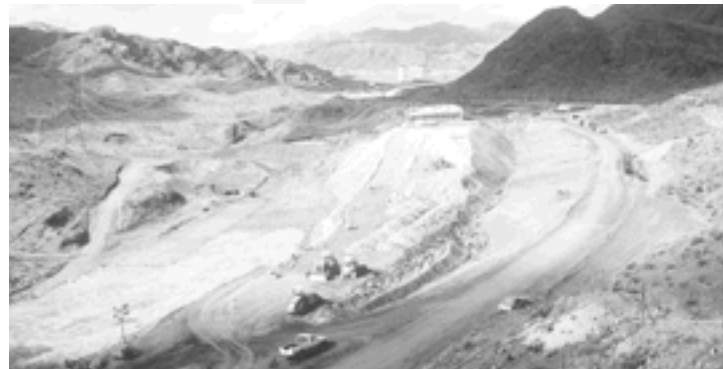
Site work progresses on the Nevada Interchange which includes ramps and a 160-foot-long bridge.
